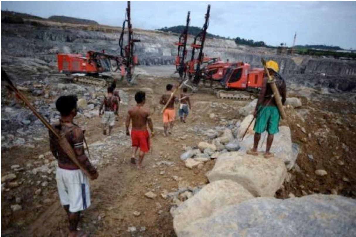
Photo 1. With 150 warriors, on May 27 2013, the Munduruku were able to take control of the immense work site at Belo Monte, controlling all of the main gates and stopping all of the activities. Photo: Lunaé Parracho.
